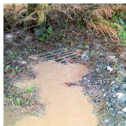
Sediment flow from roads is redirected into ponds
