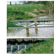
Leaky barriers made from wood
