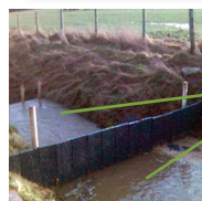
Sediment traps and a sedge wetland for nutrient pollution management
