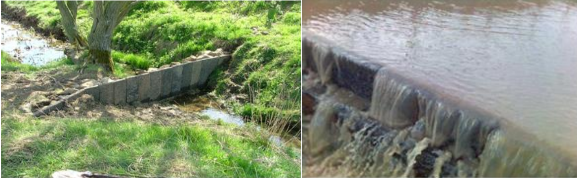
Fig. 2.7 Aquadyne barrier immediately upstream of Sedge wetland, also as seen during a storm event.
