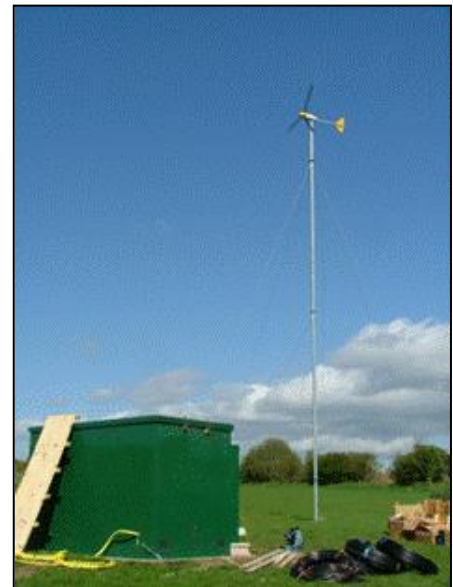
Fig. 2.2 The Green Laboratory with an Autoanalyser for telemetered on-site analysis of water quality parameters. The lab is powered by a 15m micro-wind turbine and a photovoltaic array on the roof.
