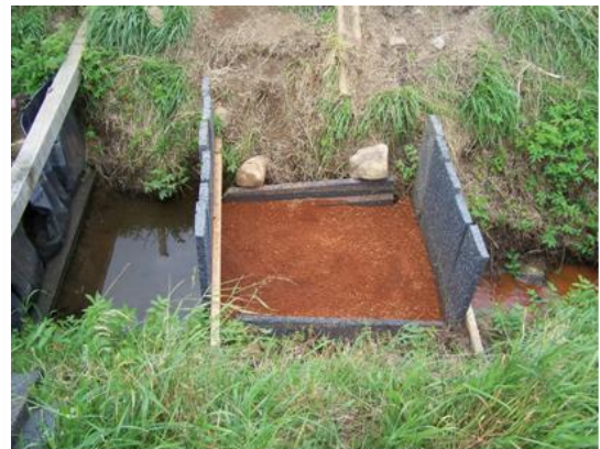
Fig 3.5 Completed ochre trap. Consists of the sediment trap upstream followed by 11 geo-textile bags, containing approximately 500kg ochre in total. Flow passes through the bags and enters a series of two ochre 'box' traps, containing collectively 860kg of ochre. The three Aquadyne dams ensure flow passes slowly through the traps and thus a high residence time is achieved.
