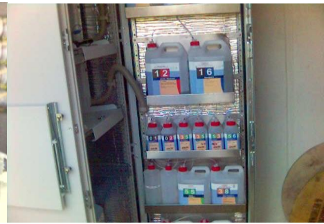
Housing of analysers with reagents for analysis
