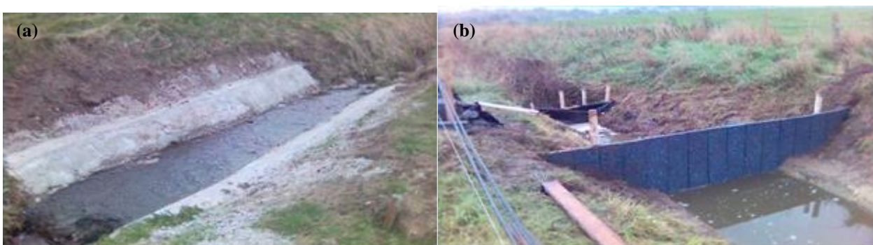
Fig.2. 5 (a) A 5-m concrete-lined sediment trap (b) trap with a barrier constructed from Aquadyne, a recycled material.
