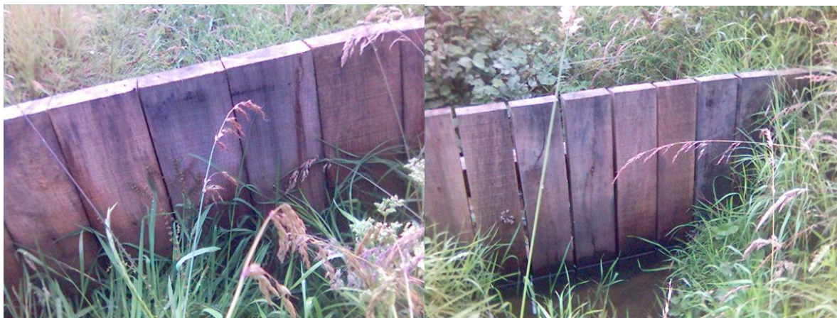
Figure 3.18, two leaky barriers, the first has small gaps between the planks, the second has 1cm gaps between the planks.
