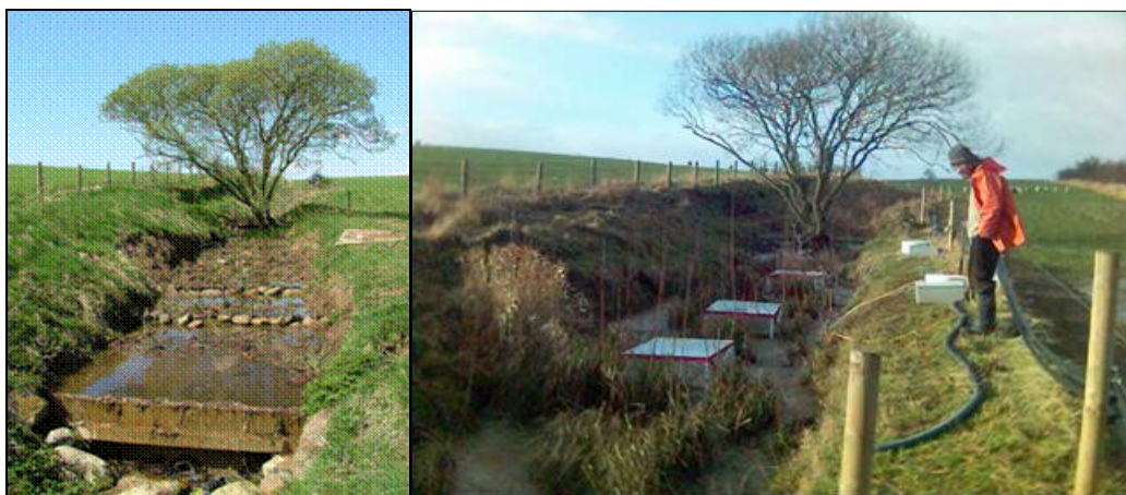
Figure 3.16. Sedge wetland after construction. Sedge is ‘borrowed’ from another local wetland to maximise denitrification in a small linear feature. Also shown are several gaseous emission chambers.
