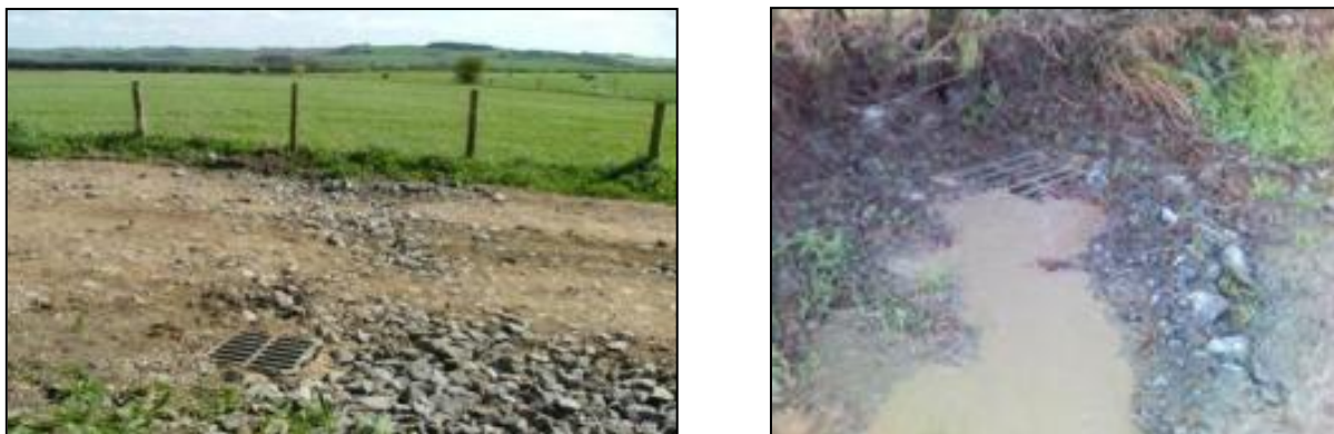
Figure 3.10. Photographs of drains that feed runoff from roads and hardstandings to the ponds
