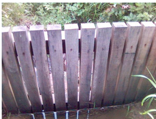
Figure 3.19, a leaky wooden barrier, with 2cm gaps.
