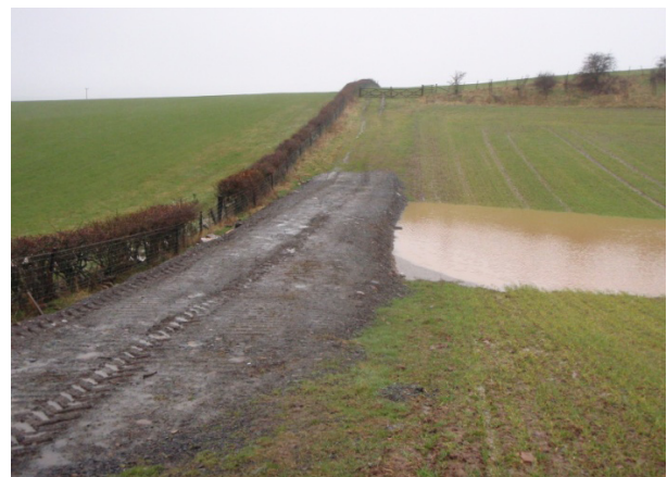
Figure 4 Bund built across a major flow pathway (base of a hollow). Left; The West Hall RAF being constructed using local soil and contractors and right; the Upper Lady's Well RAF disconnecting and storing sediment rich runoff during a storm event. This bund also acts as a road for machinery.
