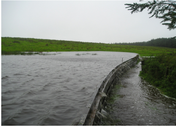
Figure 3 The pilot feature; a wooden bund disconnecting a flow pathway (left and centre: at full capacity draining slowly through the gaps in the wood and right: normal status of the feature, no disruption to farming practice).
