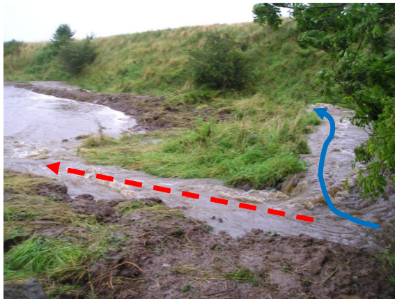
Figure 6 The simplest way to spill high channel flows into a storage feature is to lower the bank on a meander (left). However, a properly designed structure can be used in a stream to spill water out of the channel (right).
