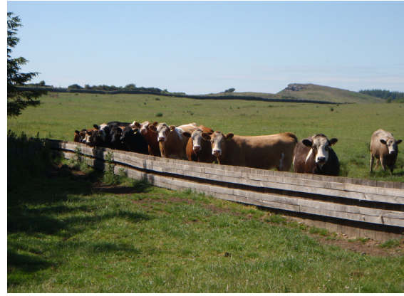
Figure 3 The pilot feature; a wooden bund disconnecting a flow pathway (left and centre: at full capacity draining slowly through the gaps in the wood and right: normal status of the feature, no disruption to farming practice).
