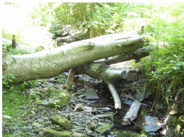
Figure 2 A woody debris beaver dam constructed in a stream with locally felled sycamore trees. Tree trunks are placed cross over to avoid bank scour
