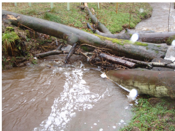
Figure 2 A woody debris beaver dam constructed in a stream with locally felled sycamore trees. Tree trunks are placed cross over to avoid bank scour
