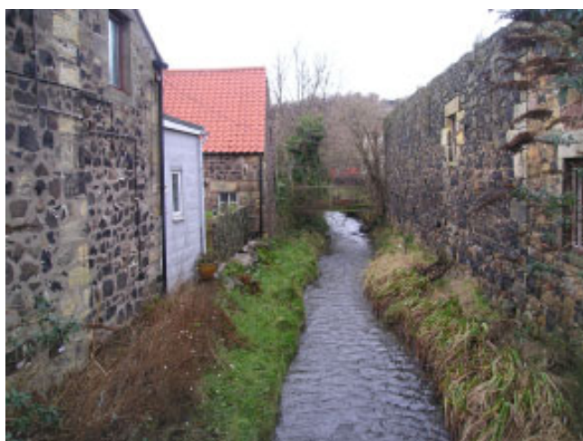
Figure 2 Belford Burn flowing through Belford. The channel is constricted between properties.
