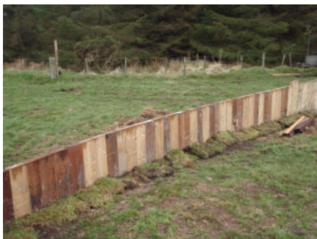
Figure 5 The wooden barrier at the bottom of the pond as it tapers out towards the hillside (to the left)
