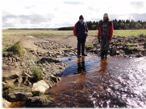
Figure 3-7 Armoured draw off channel at Dyke Head on the River Wansbeck.
