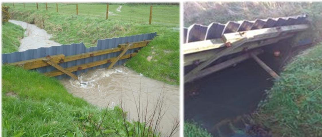
**Figure 3-6 An online plastic barrier in Hepscoth that failed during a recent flood event**
