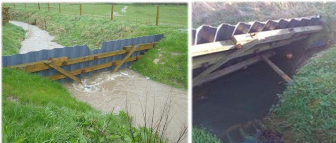
**Figure 3-6 An online plastic barrier in Hepscott that failed during a recent flood event**
