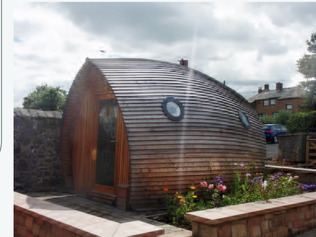
GGT, work pod, Wooler
