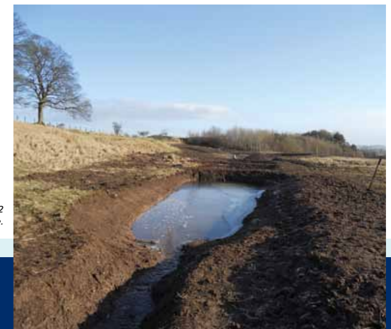
The completed works, January 2012 – inflow sediment traps and main pond feature.
