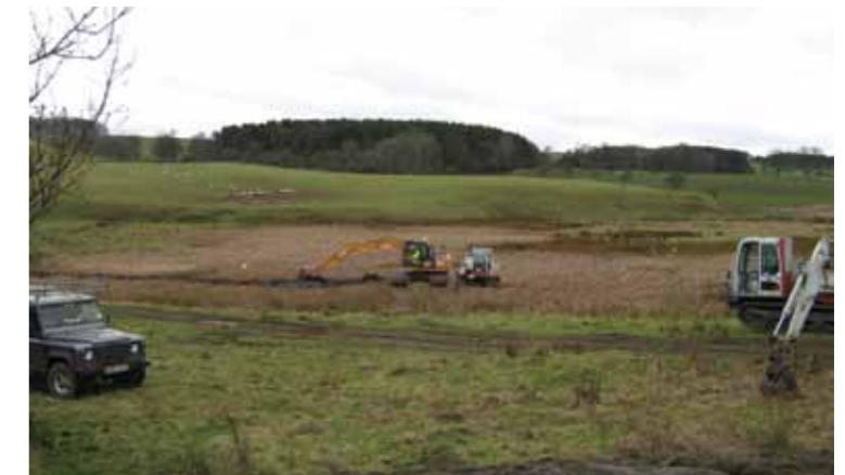
Work begins on the farm pond feature, January 2012.
