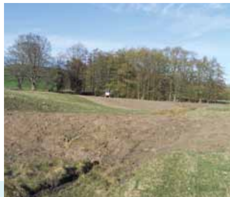
The floodplain bunds upon completion, March 2012.
